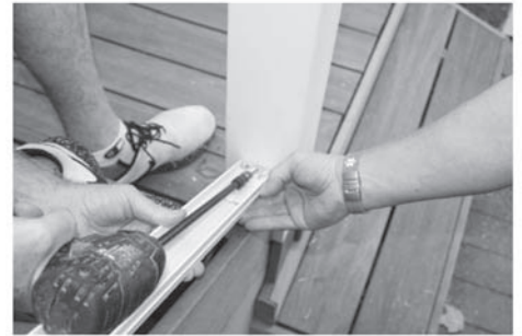
Photo 10A: DRILL PILOT HOLES FOR \frac{1}{4} " HEX HEAD SCREWS – TOP OF STAIRS
